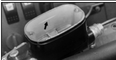
Hydraulic brake cylinder and fluid level.
